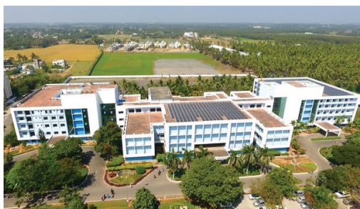
Figure 4. Solar-generation panels were installed on the roof top of the AECS building.
